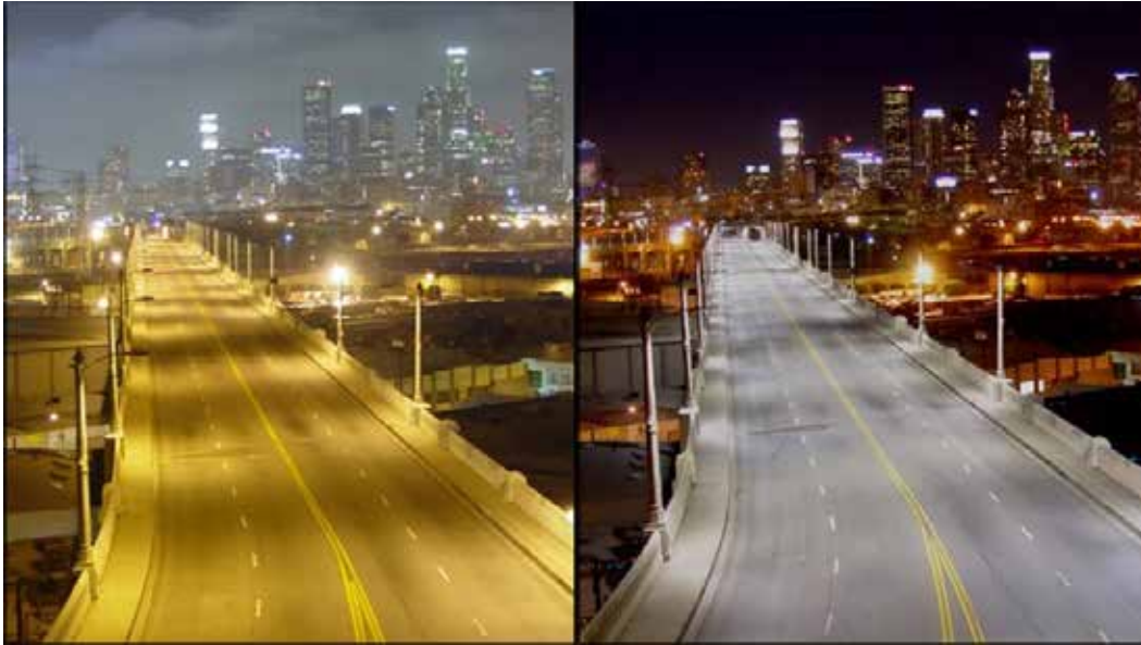
Before and after pictures of replacement lighting at the 6th Street Bridge over the Los Angeles River. The second picture shows improvements in some aspects of light pollution, as light is not directed to the sides and upwards from the upgraded fixtures, reducing skyglow. However, it also shows the use of brighter, whiter LEDs, which is not generally ideal, along with increased light bounce back from the road. Image Credit: The City of Los Angeles
